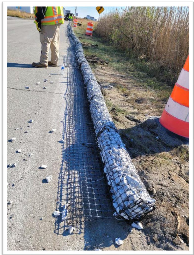
Figure 99: Installation of Fabric Wrapped Stone
